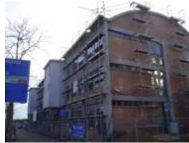
Verification of reinforcement in old buildings
